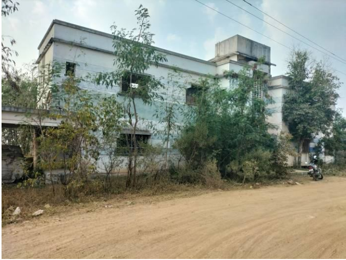
External View of Industrial Factory Shed.
