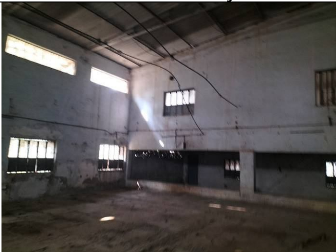
Internal View of Factory Shed.
