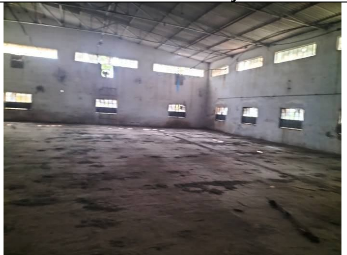
Internal View of Factory Shed.
