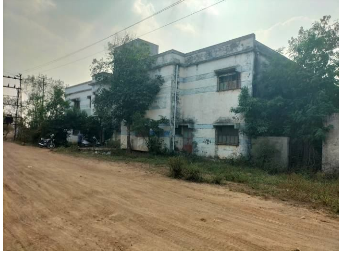
External View of Industrial Factory Shed.
